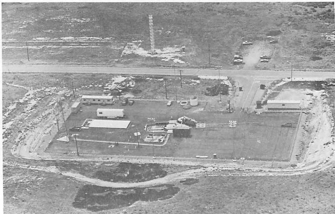
AERIAL VIEW OF PEACEKEEPER LAUNCH FACILITY 08, VANDENBERG AFB, CALIFORNIA
