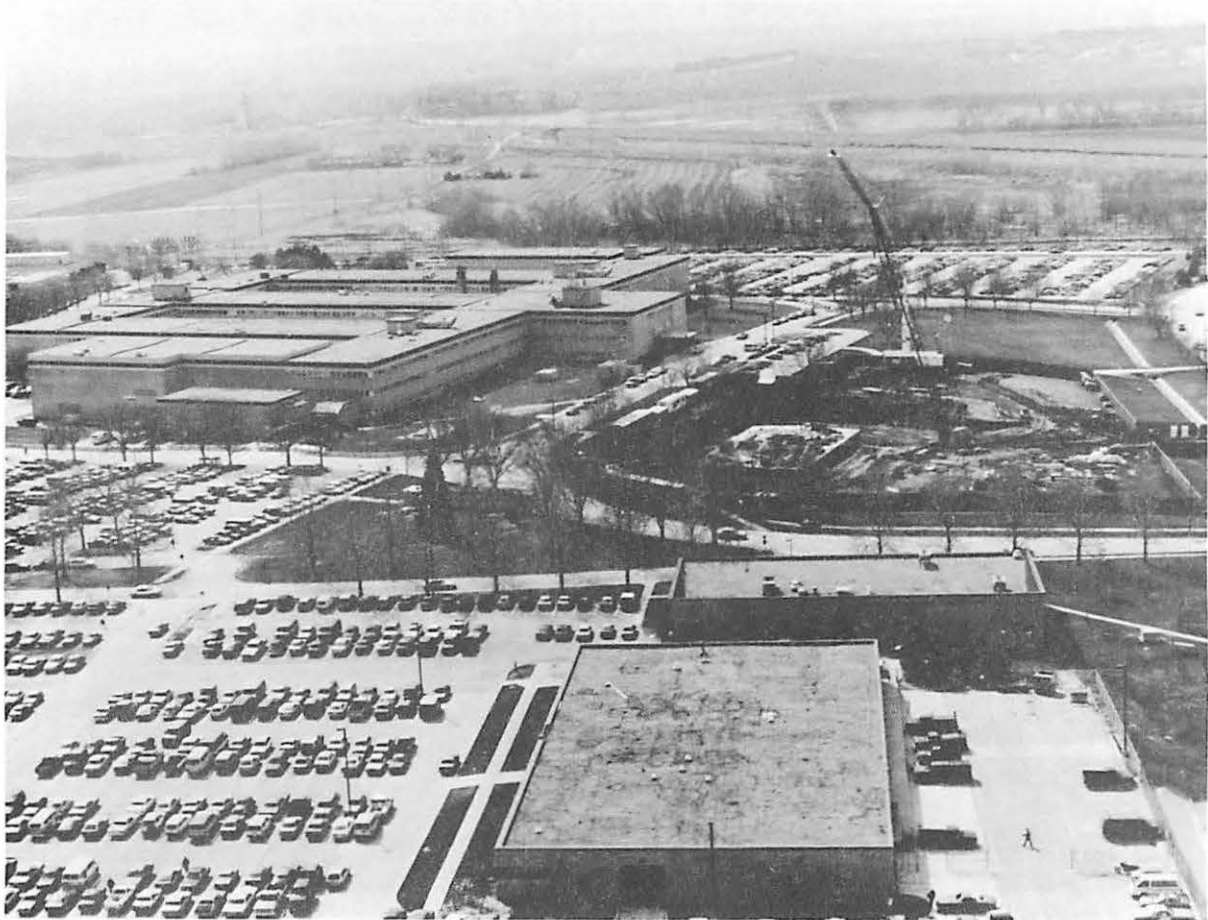
SAC COMMAND CENTER UNDER CONSTRUCTION, 1988
